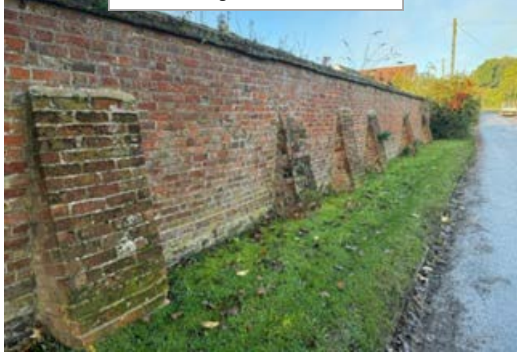
Stoke Lodge buttressed wall
